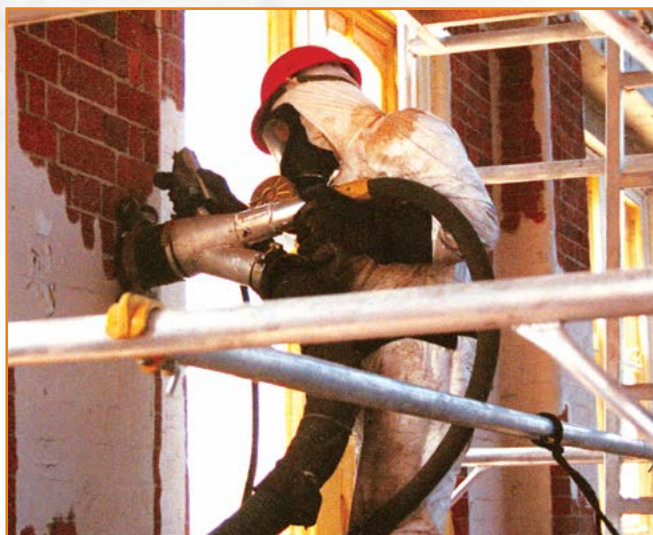
Removing hazardous paint off brickwork is made easy with the Blast 'N' Vac.
