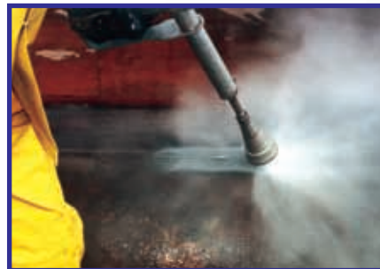
Weld inspection can be safely done with UHP water.
