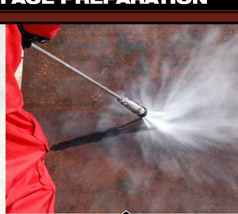
The BARRACUDA features 2 or 4 jets in controlled rotation.
